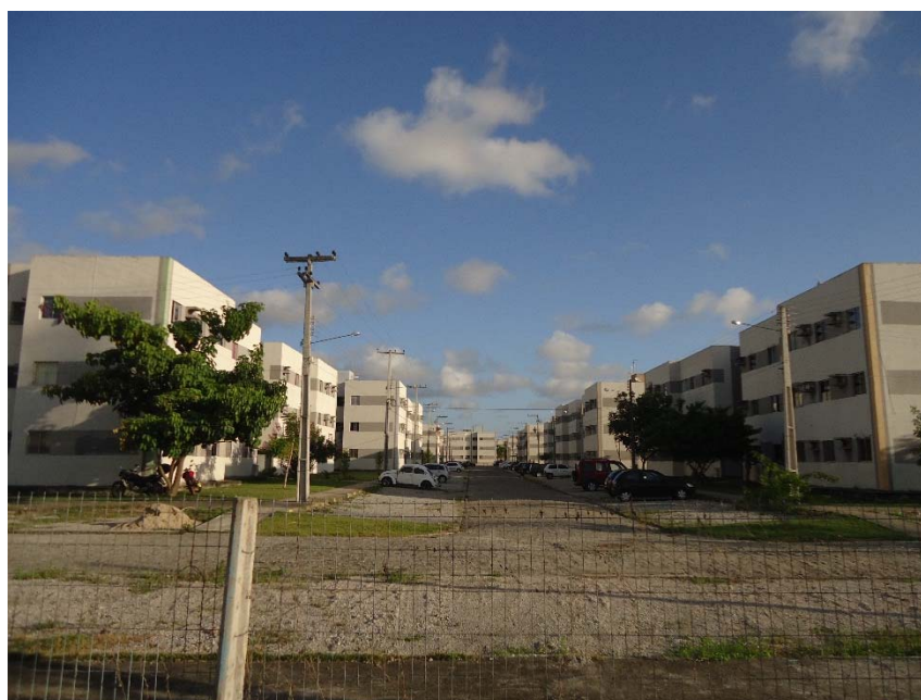
Figura 114. Condomínio Village das Artes
